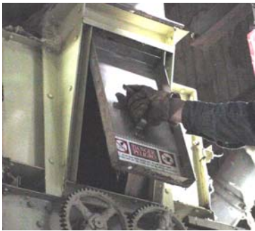
Access is provided at each end of a double entry Hopper. Inside is the cavity where dry seedcotton receives intense conditioning.
