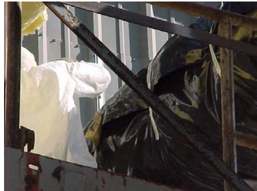
Temporarily secure film with common tape.
