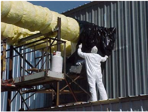
Wrap insulation with film.
