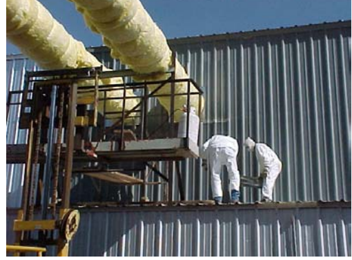
Insulation wrap complete, cut Cotton Koozie film.
